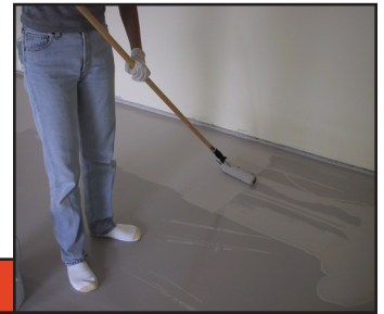
Apply using a brush and roller
