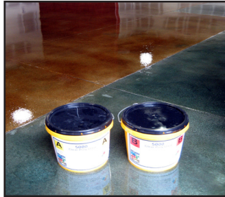
Used as a sealer over a stained floor where nearby foot traffic prevented the use of a solvenated product. Installed by Surface Solutions
