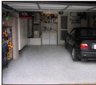
Used in residential garages
